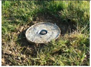
After the concrete has cured, lay in your irrigation block. Don't bother to remove the sonotube form or PVC pipe. They are fine as-is.
