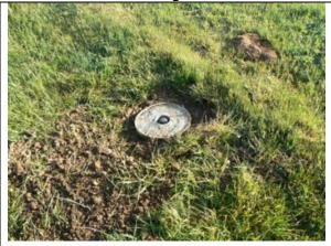
An irrigation block protects the sprinkler head and makes it easier to find.
