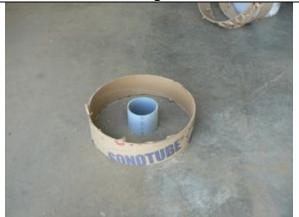
Cut a similar 3-inch slice out of a 3-inch-diameter thin-wall PVC pipe.
