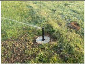
When water is flowing, the sprinkler head rises about the protective irrigation block.
