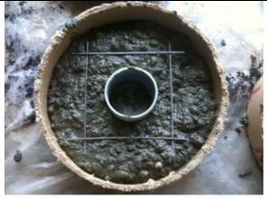
Pour the sonotune half-full of ready mix concrete. Lay the wire on top of the concrete.
