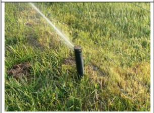
The pop-up sprinkler is buried in the ground, away from hooves, mowers, and farm equipment.
