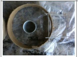
Assemble the sonotube, PVC pipe, and wire on a sheet of visqueen plastic sheeting.
