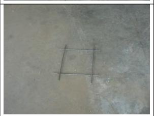
Cut a square out of 4x4 concrete wire reinforcement or hogwire fencing to fit over the PVC pipe and within the sonotube.
