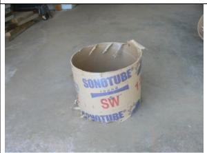
To make the irrigation block, we start with a 1-foot-diameter sonotube.
